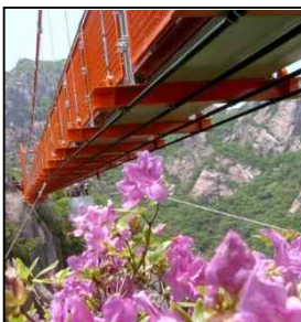
Wulchulsan Footbridge (Suspension Bridge. L=53.1m, W=1.0m. 2006). Cover of Structural Eng. International[2010.11. IABSE(Int. Ass. For Bridge and Structural Eng.)]
