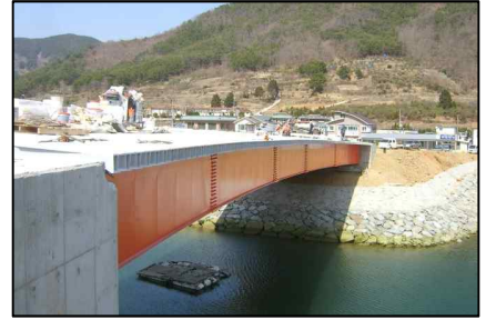
Baedoon Bridge (Steel Box Girder Bridge. L=47.0m, W=10.0m. 2009)
