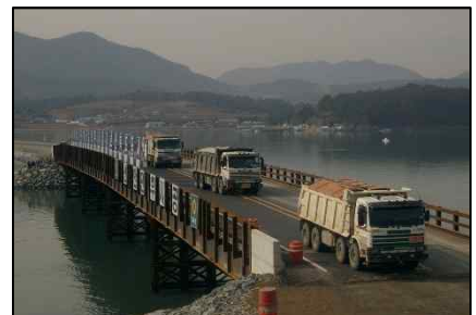
Gwangyang Bridge (Steel Plate Girder Bridge of Non-Composite Action. L=150.0m, W=10.0m. 2004)
