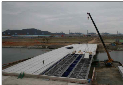
Malmoo Bridge (Steel Box Girder Bridge. L=120.0m, W=35.0m. 2013)
