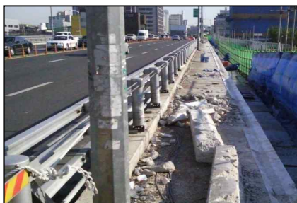
Geumchun Bridge, Walkway Expansion (PSC Girder Bridge. L=197.5m, W=3.3m. 2009)
