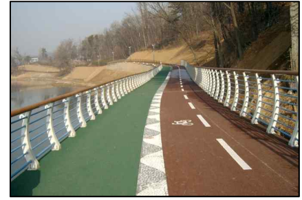
Giheung Lake Footbridge (Steel Plate Girder Bridge. L=1664.0m, W=3.5m. 2007)
