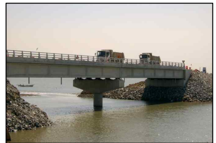
Pyungtaek Port Access Bridge (PSC Girder Bridge. L=70.0m, W=11.9m. 2008)
