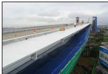
Gyulhyun Bridge, Walkway (Concrete Box Girder Bridge. Above Box Girder. L=292.0m, W=4.0m. 2011)
