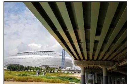
Gochuk Bridge, Walkway Expansion (Steel Plate Girder Bridge. L=406.0m, W=5.6m. 2009)
