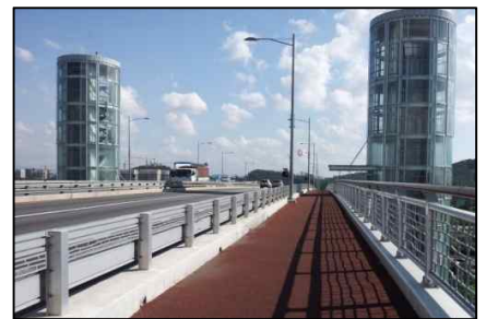
Gyulhyun Bridge, Walkway (Concrete Box Girder Bridge. Above Box Girder. L=292.0m, W=4.0m. 2011)
