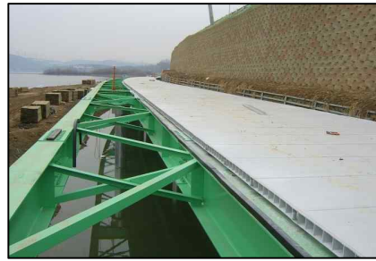
Giheung Lake Footbridge (Steel Plate Girder Bridge. L=1664.0m, W=3.5m. 2007)
