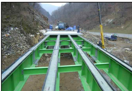
Bongsan 3-Bridge (Steel Plate Girder Bridge. L=35.9m, W=7.0m. 2007)
