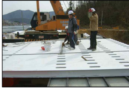
Baedoon Bridge (Steel Box Girder Bridge. L=47.0m, W=10.0m. 2009)
