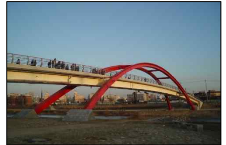
Osanshun Footbridge (Arch + Steel Box Girder Bridge. L=140.0m, W=5.0m. 2006)
