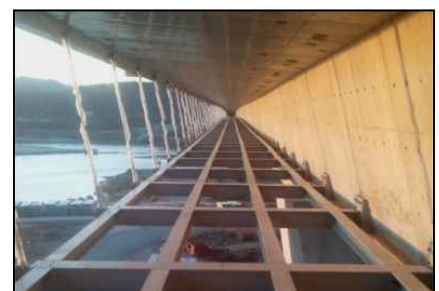
Sejong Haknarae Bridge, Walkway (Cable Stayed Bridge. Under Concrete Box. L=700.0m, W=9.0m. 2011)
