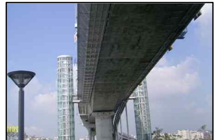
Gyulhyun Bridge, Walkway (Concrete Box Girder Bridge. Under Box Girder. L=293.0m, W=4.0m. 2011)
