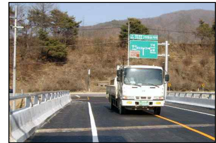
Gaejung Bridge (Steel Plate Girder Bridge. L=25.0m, W=11.0m. 2004)
