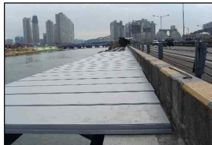
Onchun-chun Bridge, Walkway Expansion (FRP Bracket. L=144.0m, W=3.0m. 2009)
