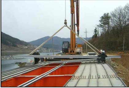
Baedoon Bridge (Steel Box Girder Bridge. L=47.0m, W=10.0m. 2009)
