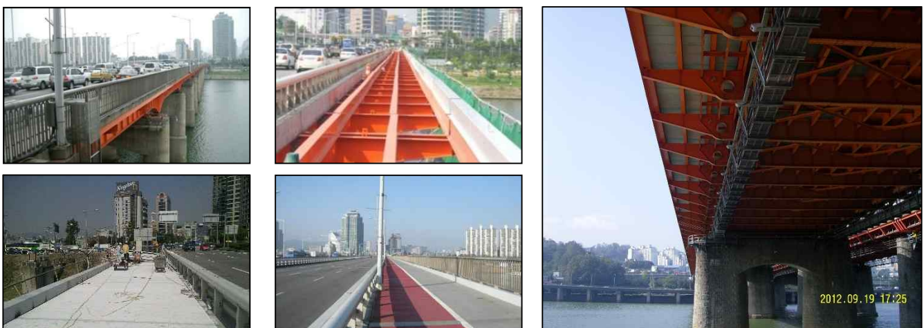
Walkway/Bikeway Expansion(Both Side) of Hangang Bridge(Plate Girder Bridge) (L=840m, W= 4.5m)
