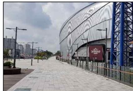
Gochuk Skydome Baseball Stadium, Walkway (Plate Girder. Walkway+Footbridge: L=410.0m, W=7.4m. 2015)
