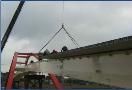
Osanshun Footbridge (Arch + Steel Box Girder Bridge. L=140.0m, W=5.0m. 2006)
