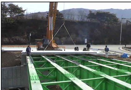
Gaejung Bridge (Steel Plate Girder Bridge. L=25.0m, W=11.0m. 2004)
