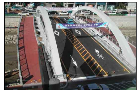
Biwoodang Bridge, Walkway (Arch + Steel Plate Girder Bridge. L=44.5m, W=9.0m. 2004)
