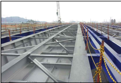
Malmoo Bridge (Steel Box Girder Bridge. L=120.0m, W=35.0m. 2013)
