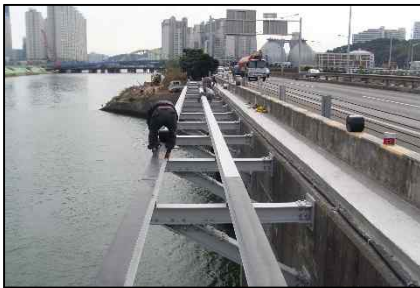
Onchun-chun Bridge, Walkway Expansion (FRP Bracket. L=144.0m, W=3.0m. 2009)
