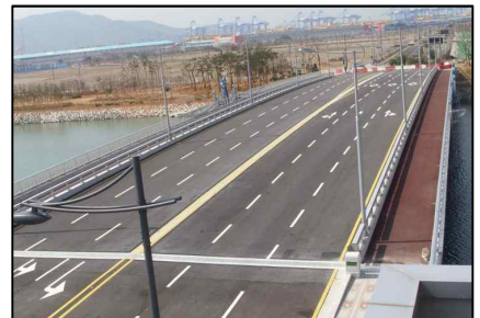
Malmoo Bridge (Steel Box Girder Bridge. L=120.0m, W=35.0m. 2013)
