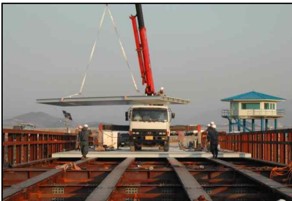
Gwangyang Bridge (Steel Plate Girder Bridge of Non-Composite Action. L=150.0m, W=10.0m. 2004)
