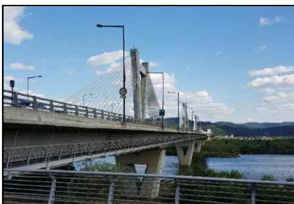
Sejong Haknarae Bridge, Walkway (Cable Stayed Bridge. Under Concrete Box. L=700.0m, W=9.0m. 2011)
