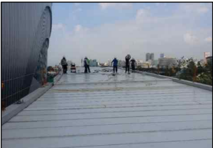
Gochuk Skydome Baseball Stadium, Walkway (Plate Girder. Walkway+Footbridge: L=410.0m, W=7.4m. 2015)
