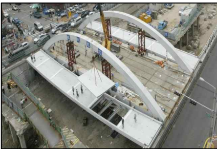
Biwoodang Bridge, Walkway (Arch + Steel Plate Girder Bridge. L=44.5m, W=9.0m. 2004)
