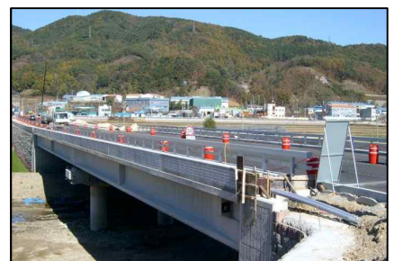
Pyungtaek Port Access Bridge (PSC Girder Bridge. L=70.0m, W=11.9m. 2008)
