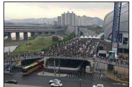
Gochuk Skydome Baseball Stadium, Walkway (Plate Girder. Walkway+Footbridge: L=410.0m, W=7.4m. 2015)
