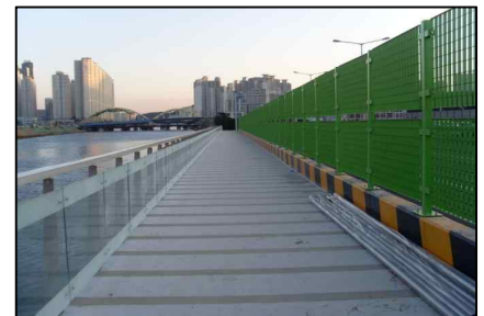
Onchun-chun Bridge, Walkway Expansion (FRP Bracket. L=144.0m, W=3.0m. 2009)
