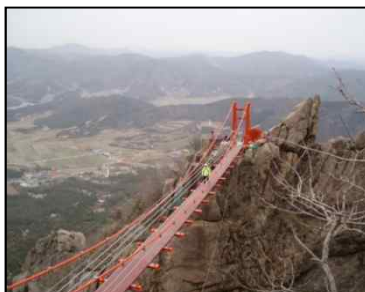
Wulchulsan Footbridge (Suspension Bridge. L=53.1m, W=1.0m. 2006). Cover of Structural Eng. International[2010.11. IABSE(Int. Ass. For Bridge and Structural Eng.)]
