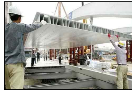
Biwoodang Bridge, Walkway (Arch + Steel Plate Girder Bridge. L=44.5m, W=9.0m. 2004)
