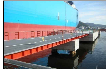
Samsung Shipyard Catwalk (Steel Plate Girder Bridge. L=82.0m, W=5.0m. 2008)
