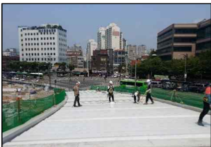
Gochuk Skydome Baseball Stadium, Footbridge [(L) Deck Installation. (M, R) Underneath View]
