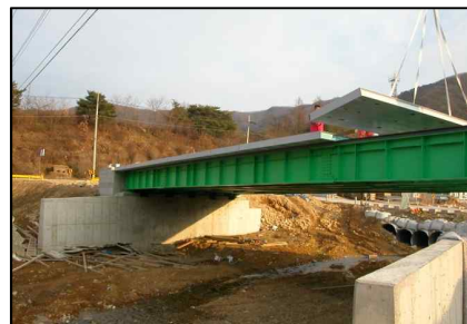
Gaejung Bridge (Steel Plate Girder Bridge. L=25.0m, W=11.0m. 2004)
