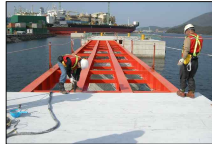
Samsung Shipyard Catwalk (Steel Plate Girder Bridge. L=82.0m, W=5.0m. 2008)
