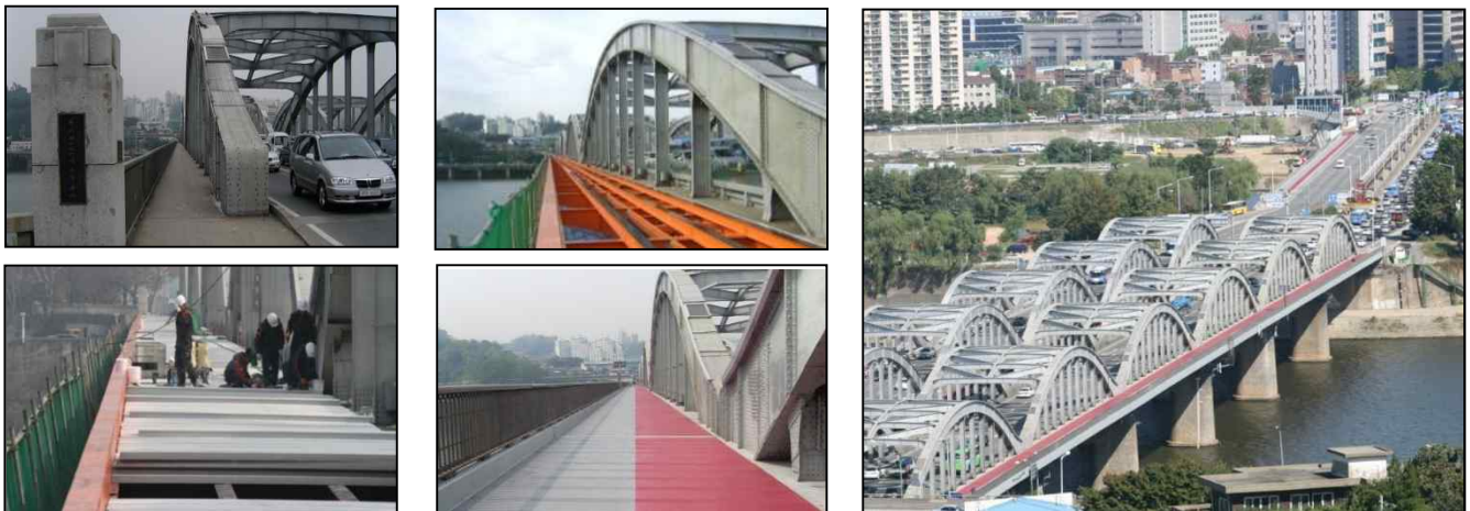
Walkway/Bikeway Expansion(Both Side) of Hangang Bridge(Arch Bridge) (L=840m, W= 4.5m)
