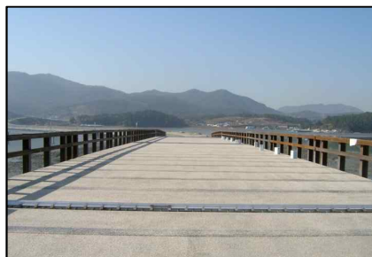
Gwangyang Bridge (Steel Plate Girder Bridge of Non-Composite Action. L=150.0m, W=10.0m. 2004)
