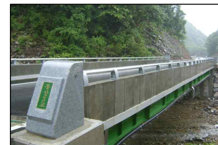
Bongsan 3-Bridge (Steel Plate Girder Bridge. L=35.9m, W=7.0m. 2007)
