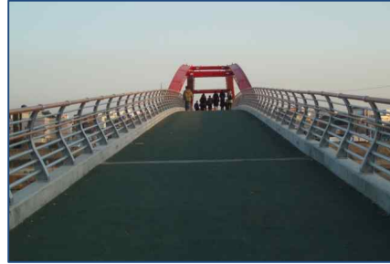
Osanshun Footbridge (Arch + Steel Box Girder Bridge. L=140.0m, W=5.0m. 2006)
